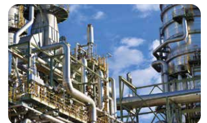
Anlagenbau | Plant construction
